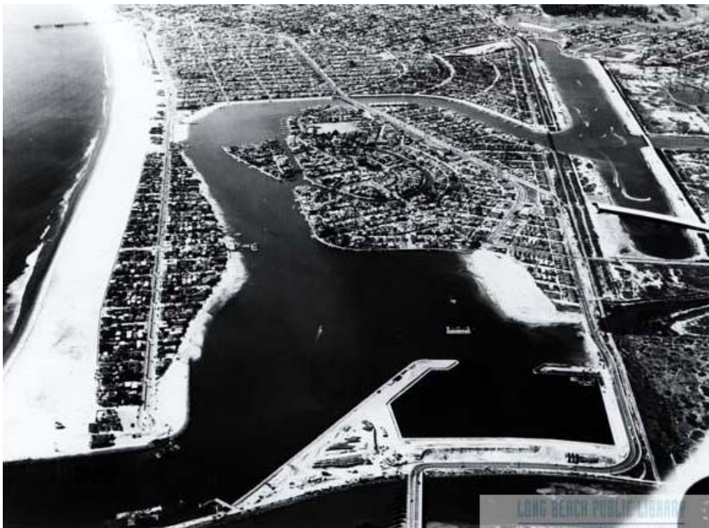
Alamitos Bay, 1956. Aerial photography shows the construction of the Davies Bridge (2 nd Street) and access to Seal Beach via Marina Drive. The Ocean Boulevard Bridge has been demolished.
